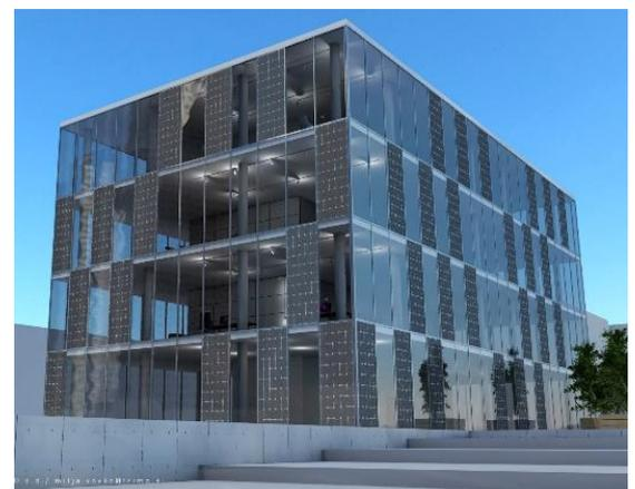
Building dimensions: 30 x 17 m<sup>2</sup>, Building ventilated volume: 7529 m<sup>3</sup>; Infiltration @ 50Pa: 0.50 ACH; U-value (Groundfloor, Roof): 0.15 W/m<sup>2</sup>K; Occupancy count: 14 m<sup>2</sup> per capita; Lightning: LED light 0.50 W/m<sup>2</sup>; Equipment: 6.00 W/m<sup>2</sup>; Internal temperature occupied days: 22 –
